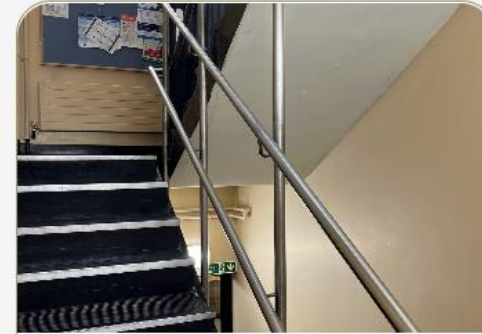
All Stairwell Balustrades
