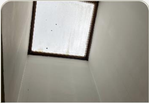
Plasterboard to rooflight wells
